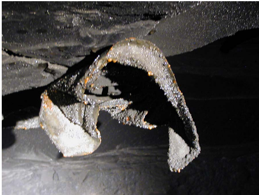
Photo 6. An example of a severely deformed roof pan (“spider plate”) that was found in the #9 entry just inby Seal #10. This is typical of the degree of bending and damage found between the seals and just after the first line of crosscuts inby the seals. This type of damage was also found in other areas of the mine where there were significant obstructions and where there was first-mining only (no “bottom-mining” done on retreat).
