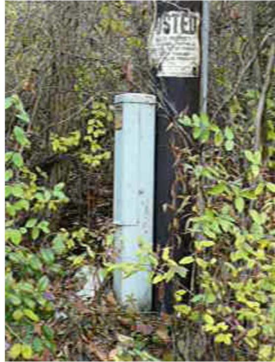
Photo 15: Junction box of 1981 line - where line changes from aerial to buried
