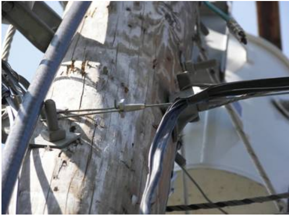
Photo 21: Messenger wire on new line (not grounded on pole)
