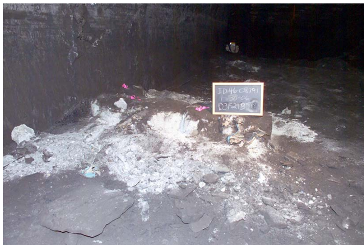
Photo 3. Location: Seal #2 (Courtesy of MSHA)
