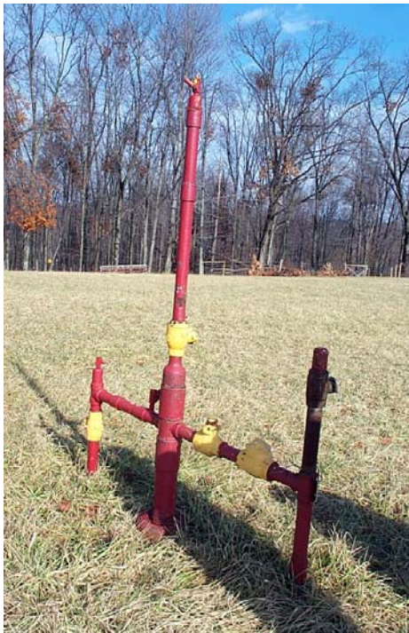
Photo 12. Nearest known gas well to the Old 2 nd Left Section. Soil resistivity tests were conducted here.
