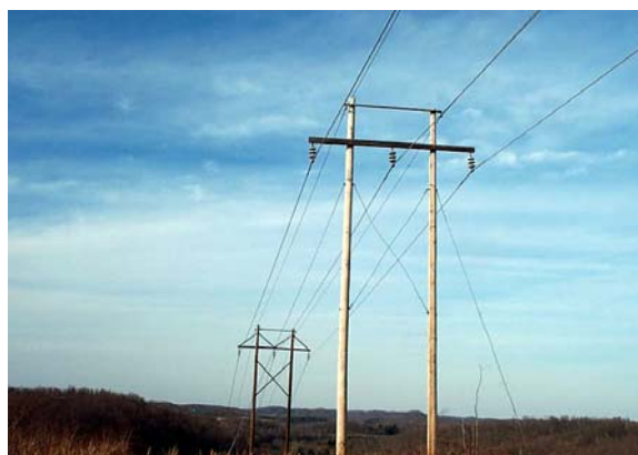
Photo 5. Section of 2.6 mile 12KV power line
