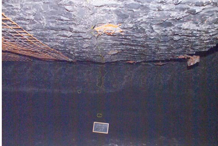
Photo 8. Location: Seal #7 (Courtesy of MSHA)
