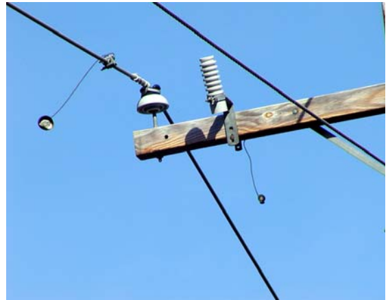
Photo 9. Damaged lightning arrester on the outside phase of the branch line feeding the Sago sub-station
