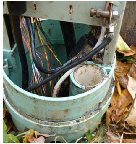
Photo 17: Typical grounding of buried cable at junction box
