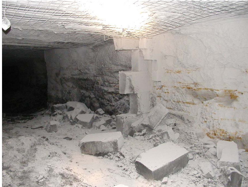
Photo 10. Remnants of a stopping in an area outby the seals.
