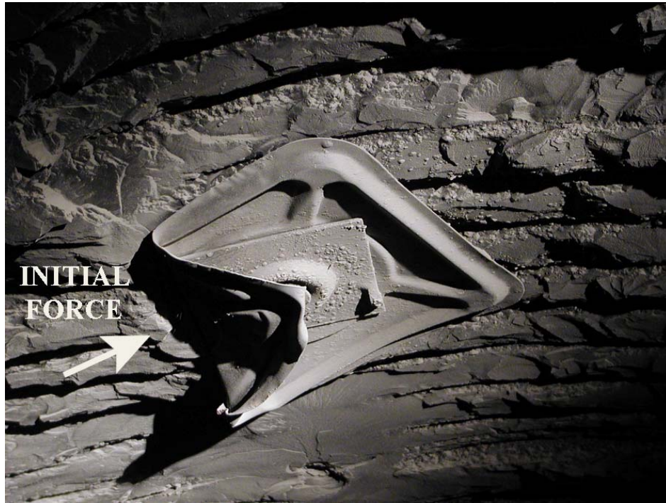
Photo 3. Simple plate bending of a roof pan in one direction. When neighboring pans also showed bending in the same direction this was plotted on the Flames and Forces Map as a single black arrow.
