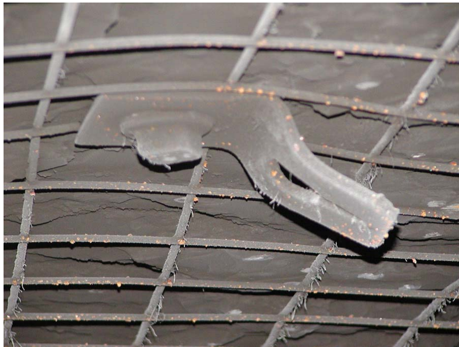
Photo 7. An example of a bent belt hanger, which were usually bolted directly to the mine roof with no pan underneath. Their purpose is to provide an anchor point to hook chains to suspend the conveyor belt structure. This is a smaller version of the 4" x 4" belt hanger flanges that were typically used throughout the mine. Originally the angle of the flange was 90° (+/- 1 degree). This bending was studied as another source of information to interpret blast force direction and magnitude.
