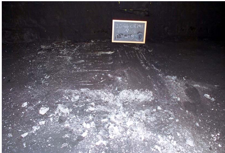
Photo 5. Location: Seal #4 (Courtesy of MSHA)
