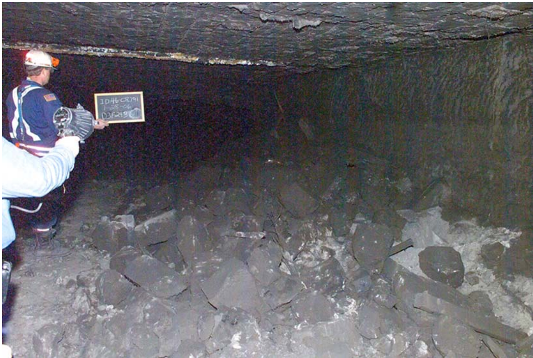
Photo 1: Omega Debris - In First Outby Crosscut Between Seal #1 & #2 (Courtesy of MSHA)
